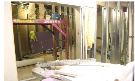
Work Begins on New Nurse Care Bays Near 400 Hall
