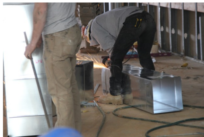
Welders Prepare New HVAC Duct Work
