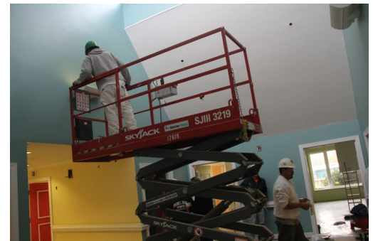
Painting Crews Finish on 600 Hall
